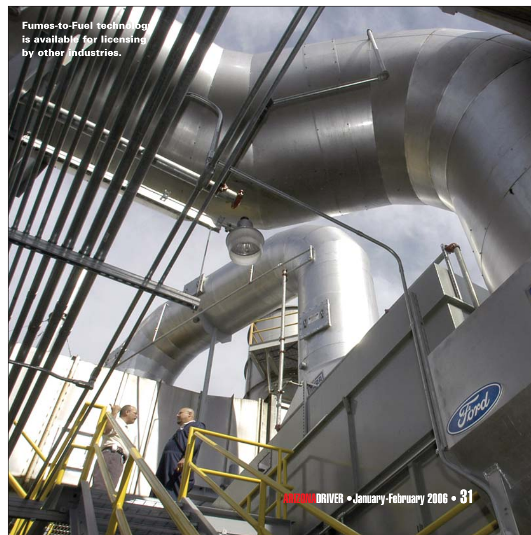
Fumes-to-Fuel could save one-third to one-half the cost of traditional incineration of volatile organic compounds (VOCs).
